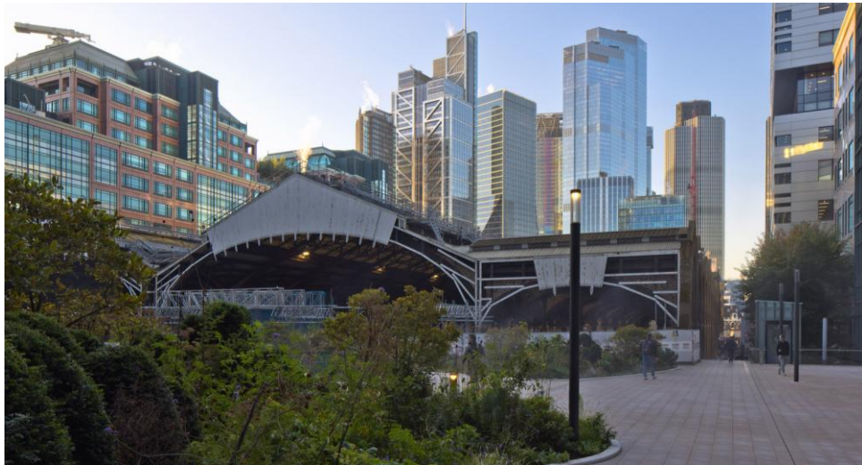
Rear elevation of Station and Exchange Square
