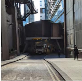
1 - Ramp from Primrose Street
